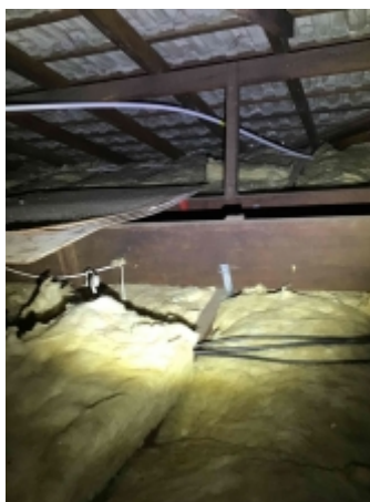
Parts of the roof space due to accessibility
