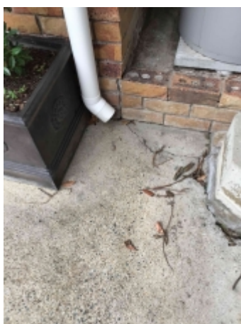
Showing example of downpipes
