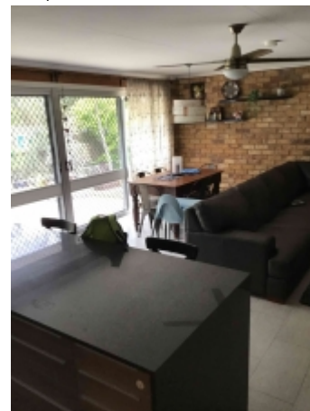
Showing examples of obstructions (e.g. wall, floor, ceiling coverings, cabinets, window furnishings, vegetation, insulation and ducted AC, furniture and stored goods, etc.)
