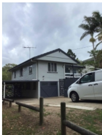
Upper roof due to accessibility
