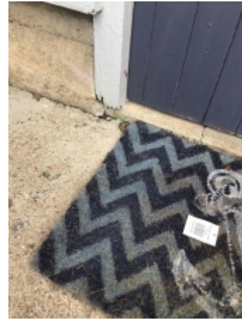
Showing example of bridging
